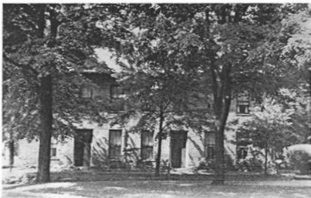
The Griswold Tavern, erected in 1811, is one of Worthington's most historic homesteads.
