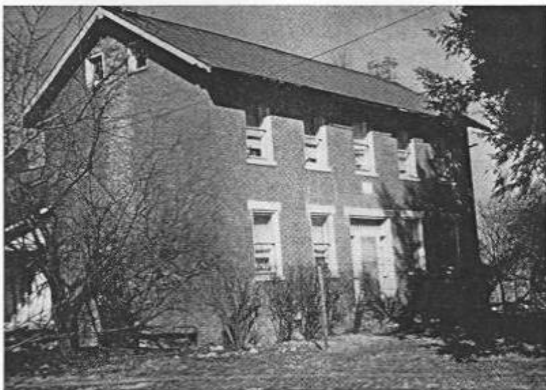
William Whims burnt the brick for this homestead in his own kilns.
