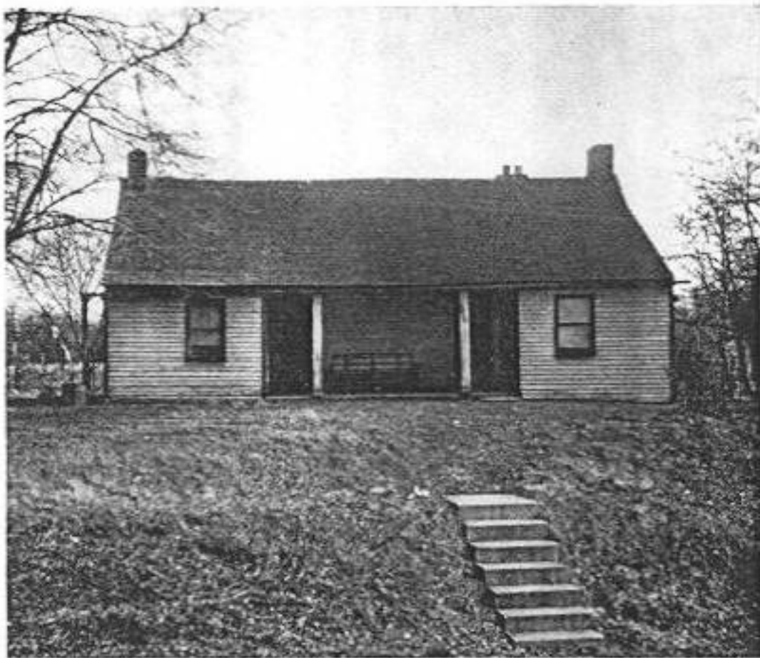
A recessed porch with flanking pavilions all pulled together by a low-pitched hip roof make this a unique farm house.
