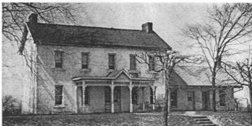
This homestead, built by David Spangler in 1815, is the oldest structure of any kind in Franklin County south of Columbus.
